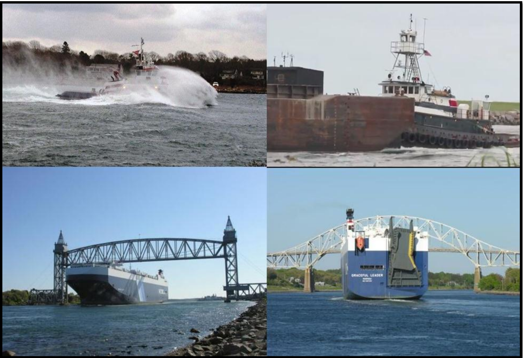
Attachment 1b. Various vessel traffic in Cape Cod Canal including turbulence at entrance and large car carrier approaching bridges
